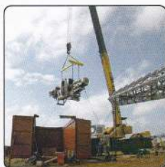
Assemble of the nacelle
